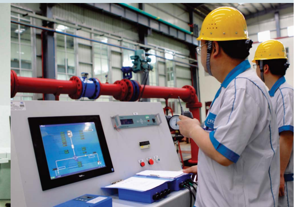
Testboard for small and medium-sized pumps
