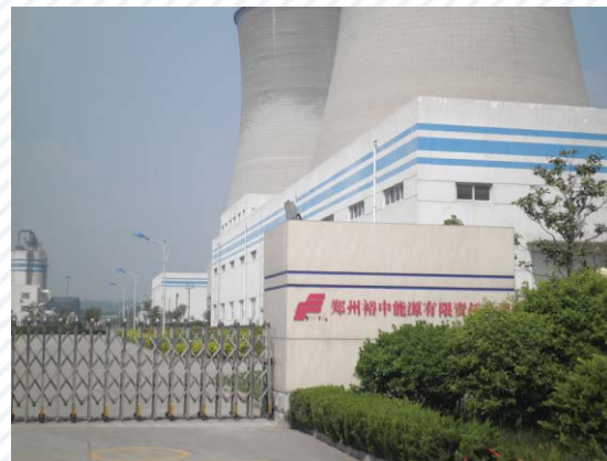
Zhengzhou Yuzhong Energy LLC Xinmi Power Plant Phase II Circulation pump 2X1000MW
