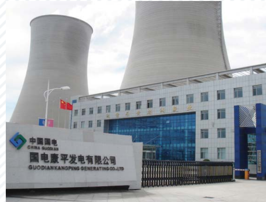
Guodian Kangping Power Generation Co., Ltd. Circulation pump 2X600MW
