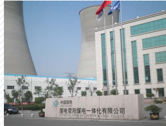
Guodian Xinyang Coal-electricity Integration Co., Ltd.
